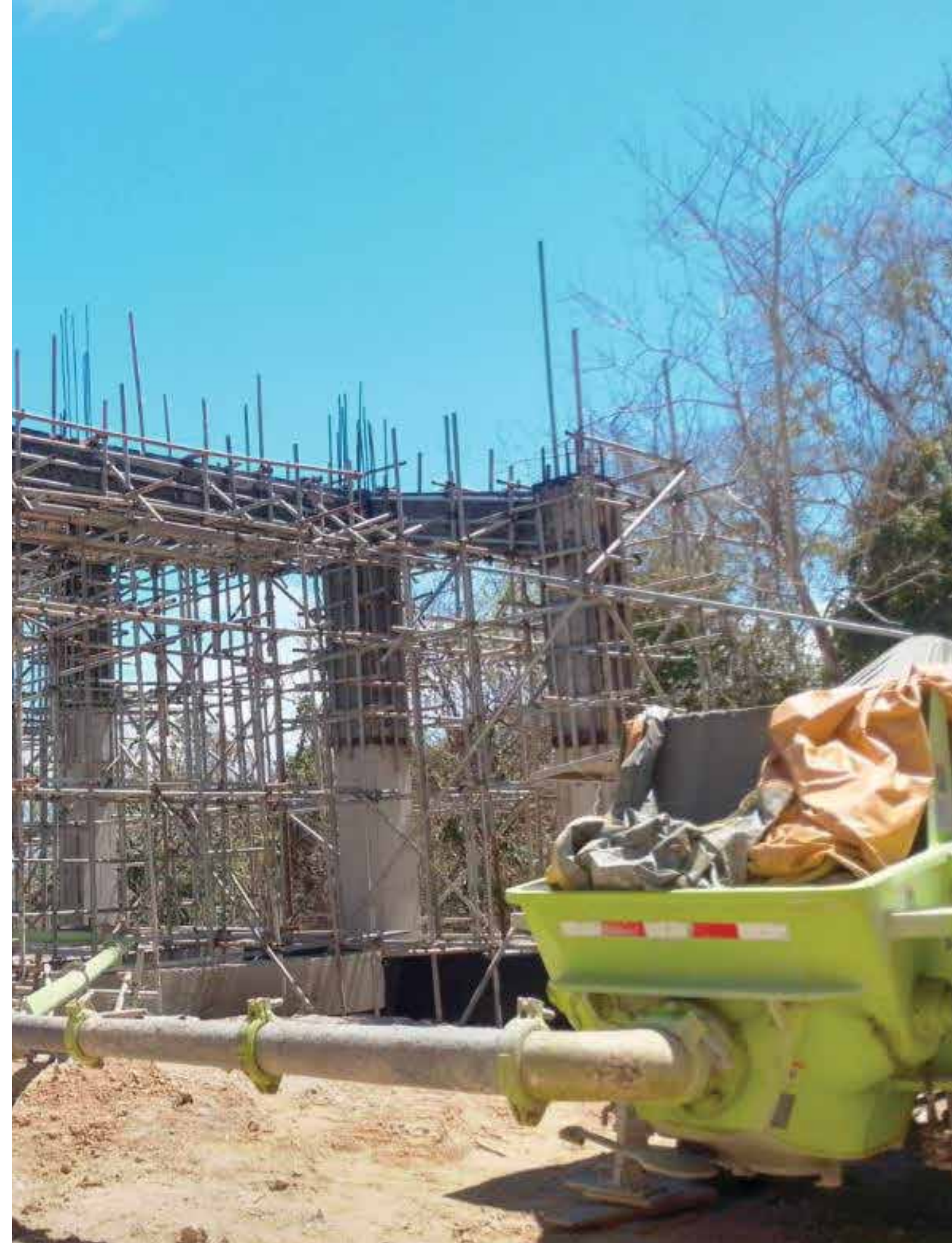
Preparation For Concrete Pouring
