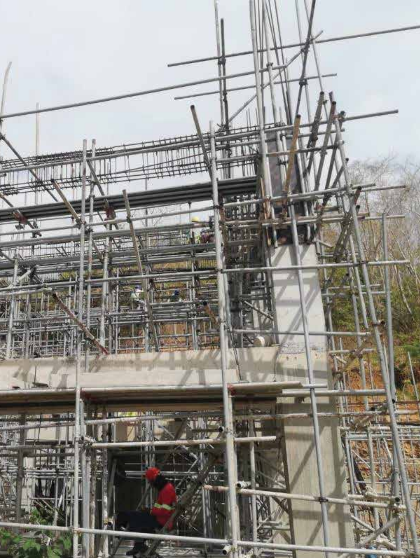
Installation Of Forms
