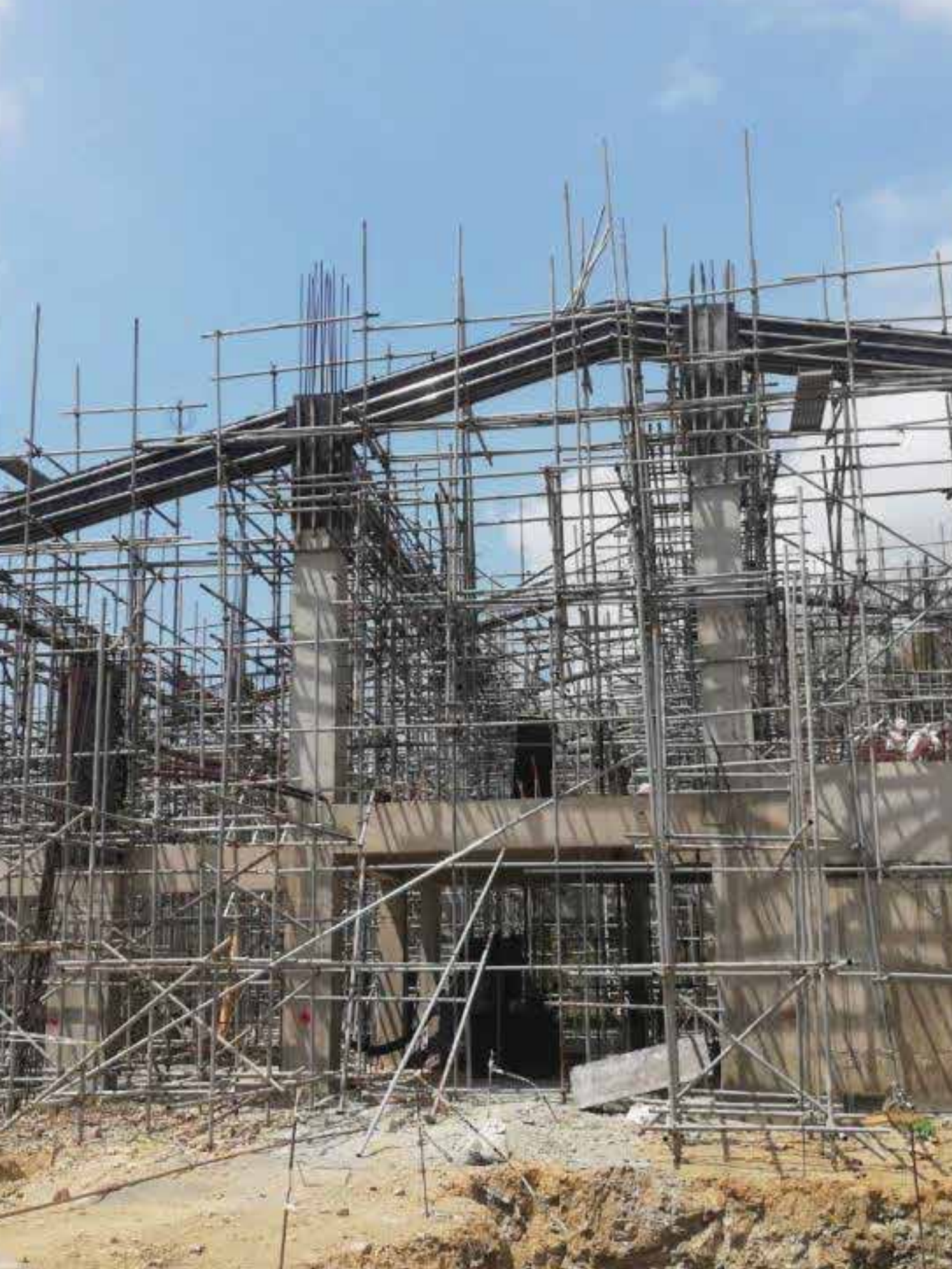
Erection Of Suppports & Scaffoldings
