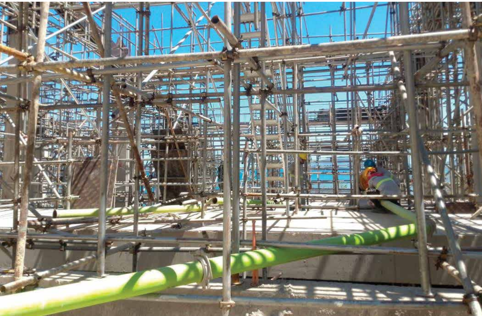
Pipe Laying For Concrete Pouring
